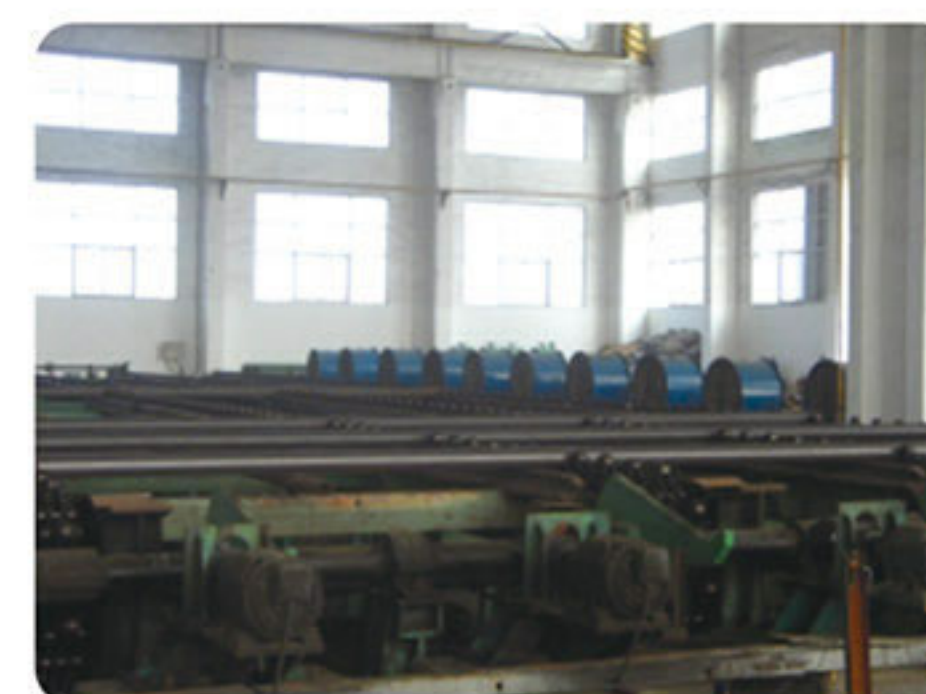
Cooling bed Stepwise cooling bed, lifted by motor-transmitted, hydraulic-controlled translating, cooling sectioned as 27*28m, dual-feeding available.
