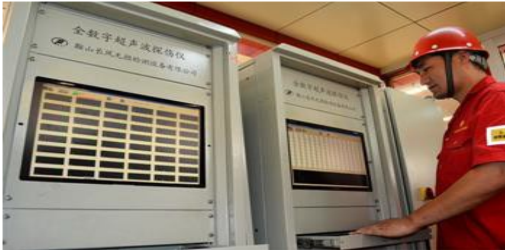
Continuous Monitoring Equipment of Ultrasonic Flaw Detection
